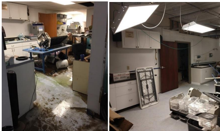
Figure 4. SNC "Orbiculture lab" immediately after flood (left) in August 2018 and in process of renovation (right) March 2019.
