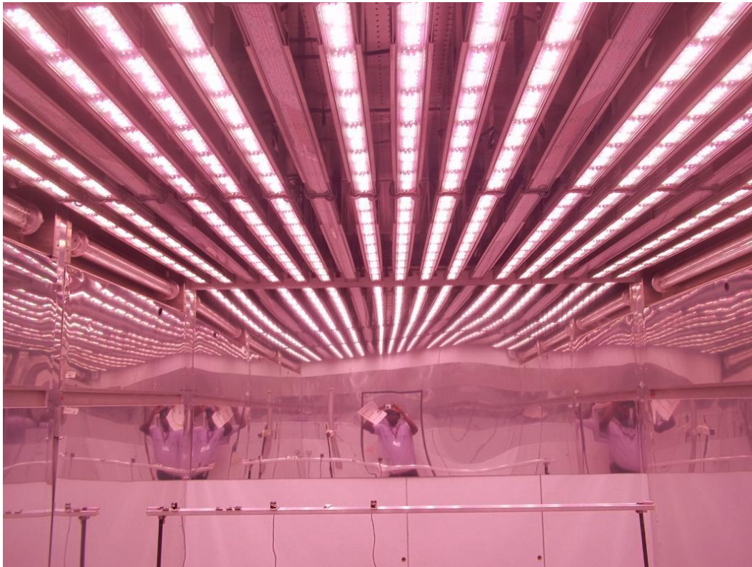
Figure 1 - Interior of BDW120 with Valoya LEDs
