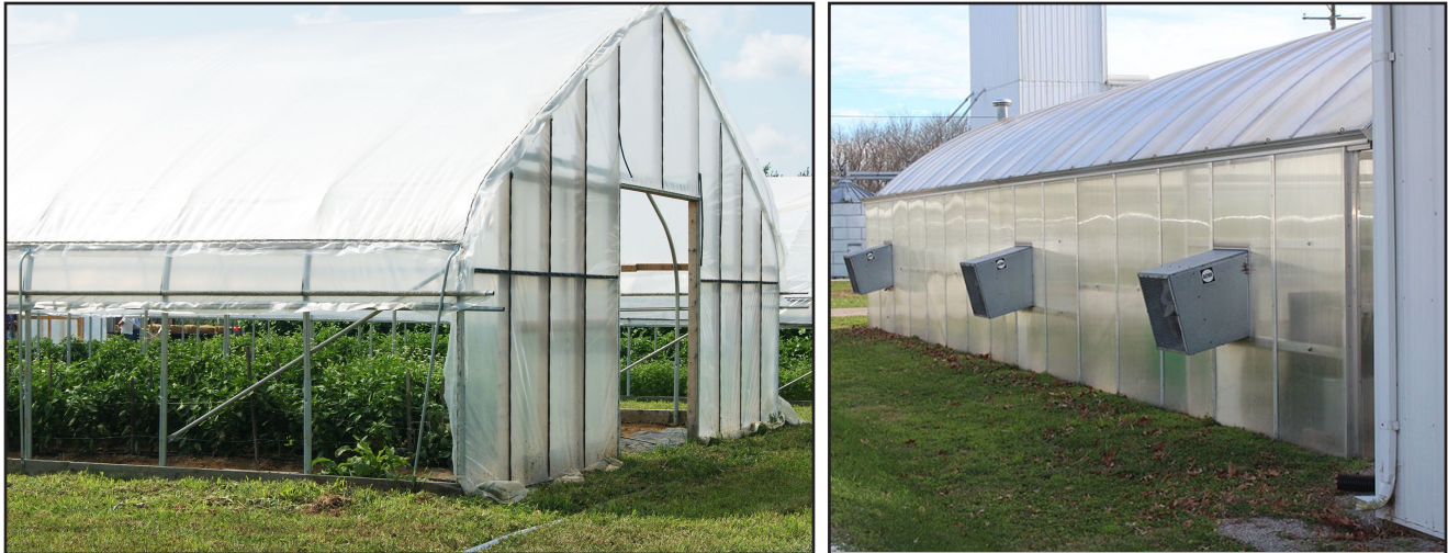
FIGURE 2. VENTILATING HIGH TUNNEL (LEFT) AND GREENHOUSE (RIGHT) STRUCTURES IS IMPORTANT TO REDUCING INTERNAL RELATIVE HUMIDITY. HIGH HUMIDITY ENCOURAGES THE DEVELOPMENT OF MANY DISEASES, SUCH AS POWDERY MILDEW AND BOTRYTIS GRAY MOLD.
