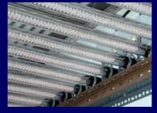
Figure 5. LED arrays mounted inside a CE room
