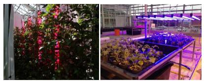
Figure 1. ORBITEC greenhouse supplemental lighting systems. LED in-canopy light tower at Purdue University (L). LED light bars assembly at University of Tennessee (R).
