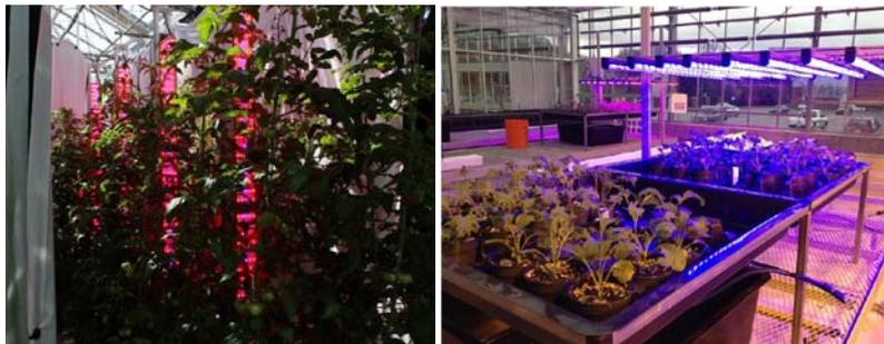
**Figure 1. ORBITEC greenhouse supplemental lighting systems. LED in-canopy light tower at Purdue University (L). LED light bars assembly at University of Tennessee (R).**
