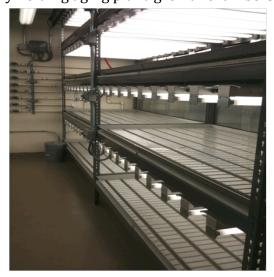
small louvers on each shelf. The room is kept under positive pressure, and door sweeps and Mars air-curtain doors installed to reduce pest flow into the room. Alarms are installed to turn off power in the event of high air temperature or flooded floors.
