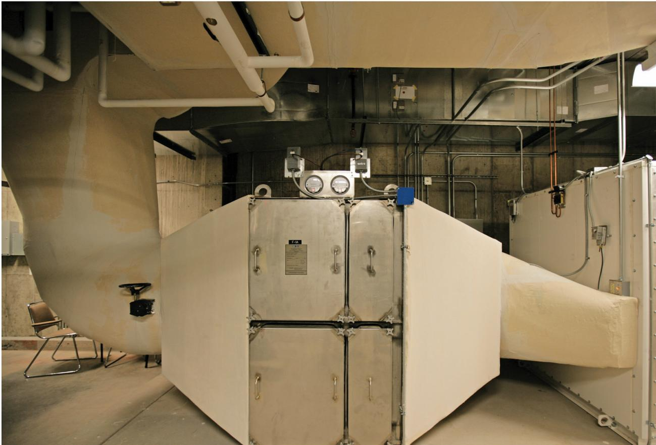
**FIGURE 15. Bag-In, Bag-Out HEPA Filter System Attached to Air Handler\***
