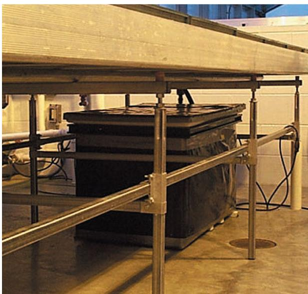
**FIGURE 17. Ebb and Flow Bench with Collection Tank**
