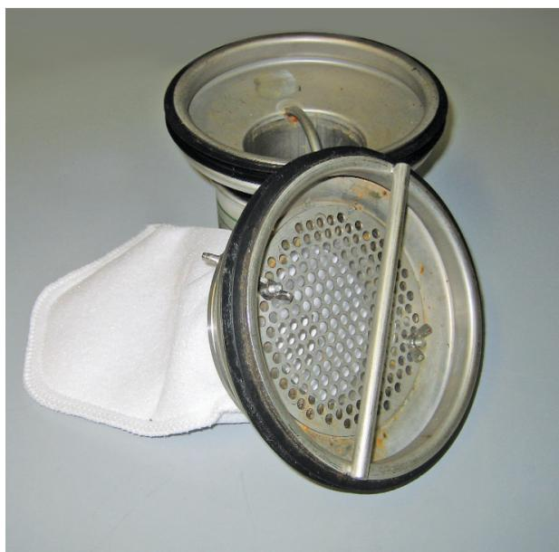
**FIGURE 11. Filter Sock on Floor Drain\***
