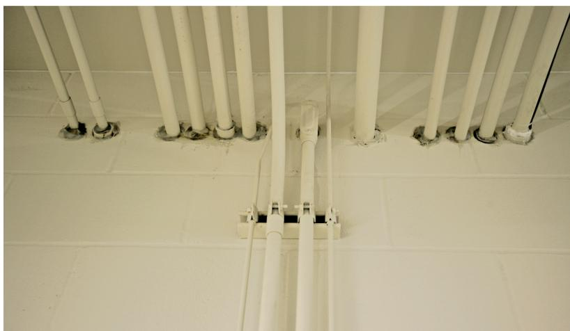
**FIGURE 18. Caulking around Service Intrusions\***
