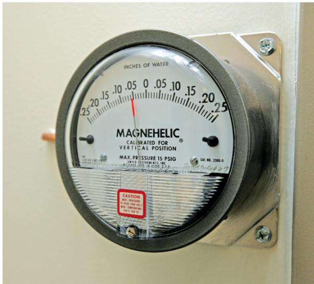
**FIGURE 16. Magnehelic Gauge for Visual Confirmation of Pressurization**
