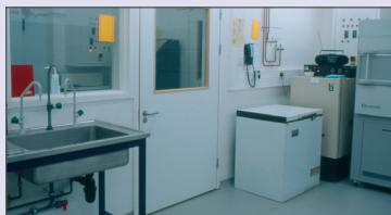
The whole area is a sealed unit entered through a double door system, all internal doors are fitted with alarms to prevent any two adjacent doors being opened at the same time
