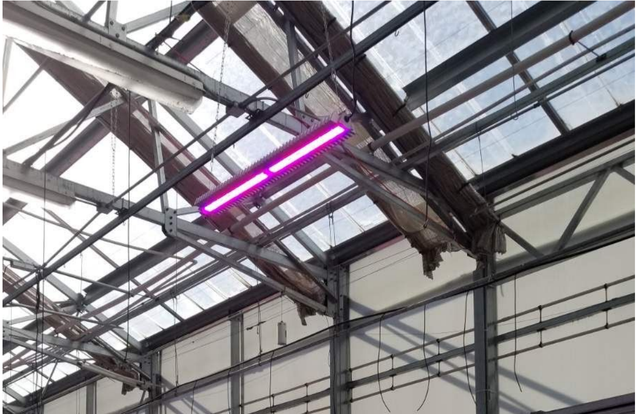
Installation of new high-output LED grow lights. (L1000 supplied by GE)
