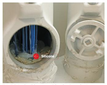
FIGURE 1. Caulking around Service Intrusion\*
