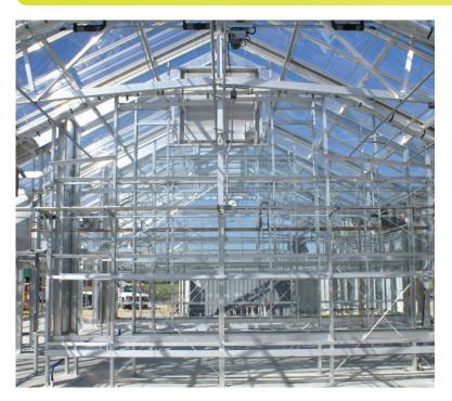
FIGURE 9. Aluminum Framing\*
